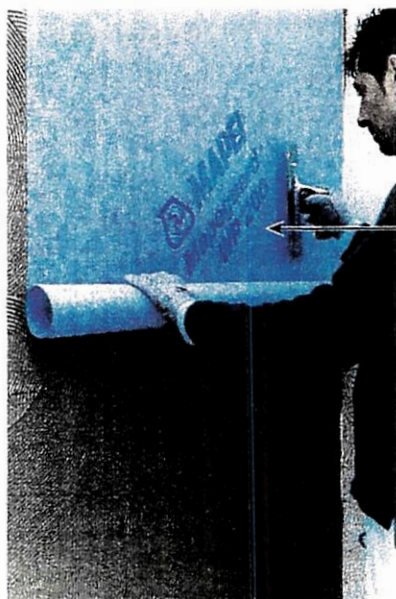
Figure 1.17 Pose de membrane
