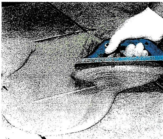
Figure 2.12 Application du coulis
