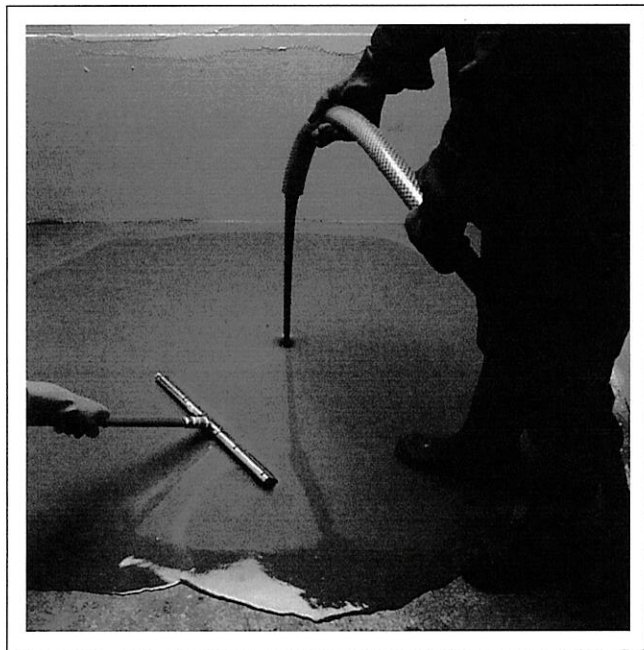
Figure 38 Coulis de ciment (Mapei) (Novo/Plan 2)
